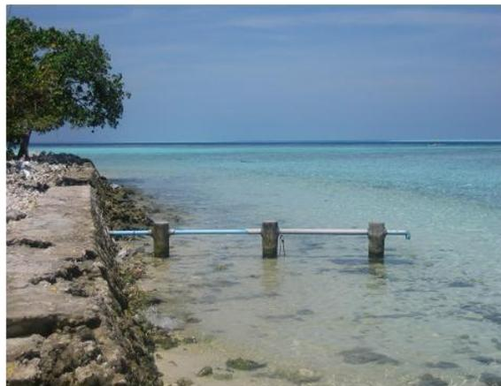
Sewer outfall of small bore sewerage system, K. Gulhi (Photo: Mustafa, 2006)
